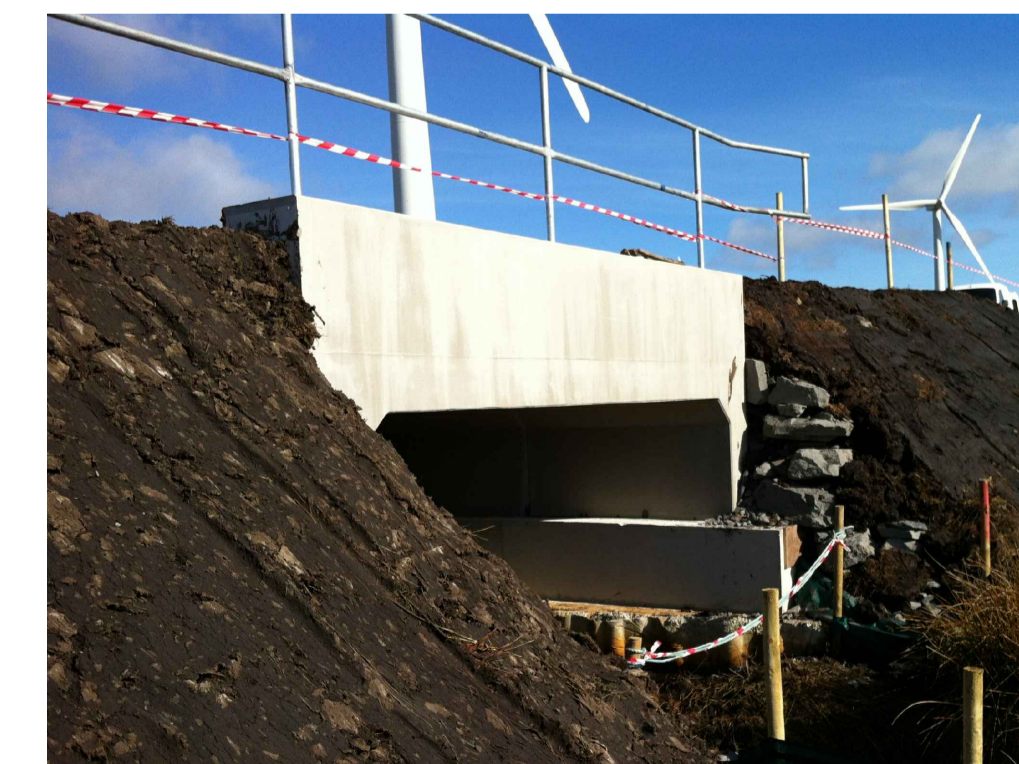
Bottomless Box Culvert Crossing
