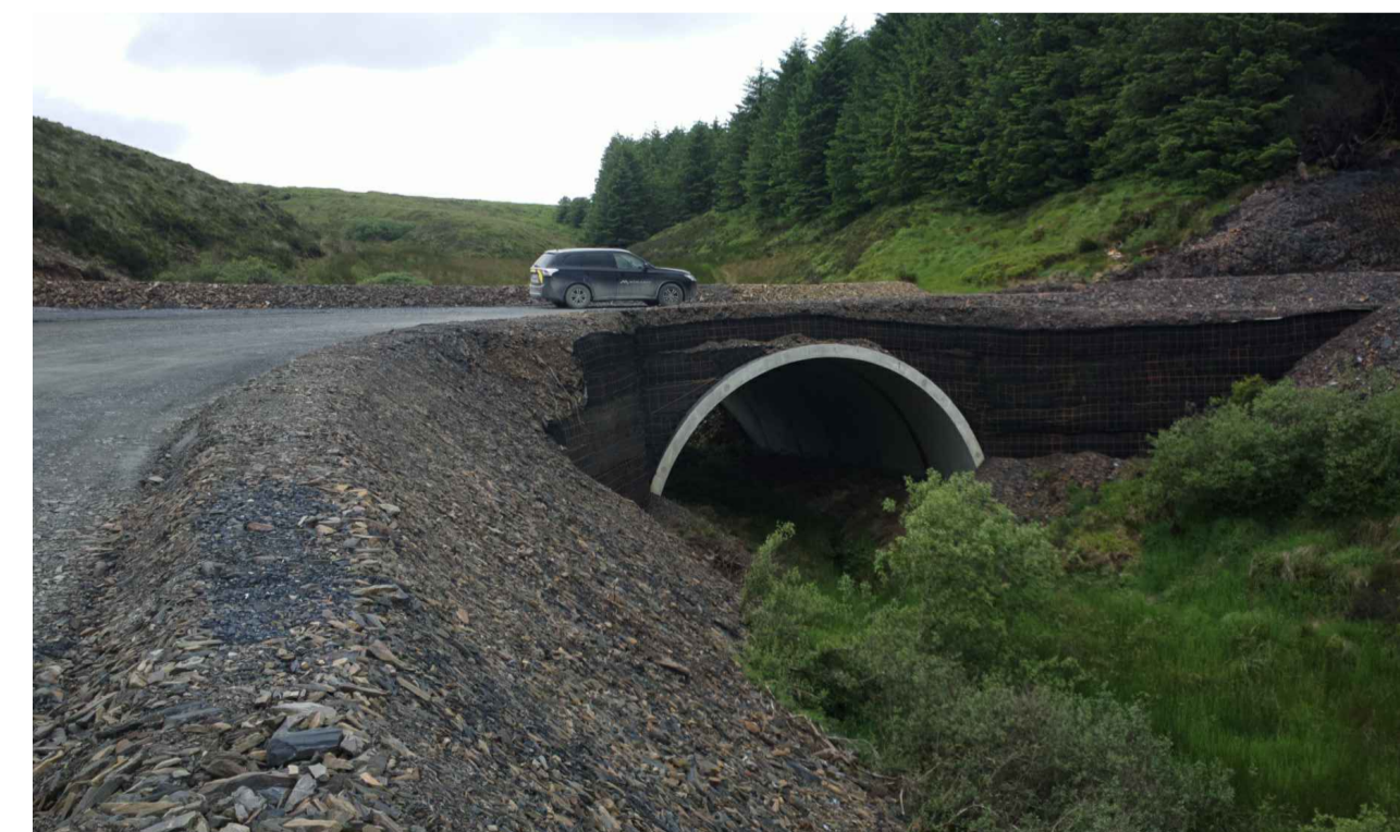
Bottomless Arch Culvert Crossing
